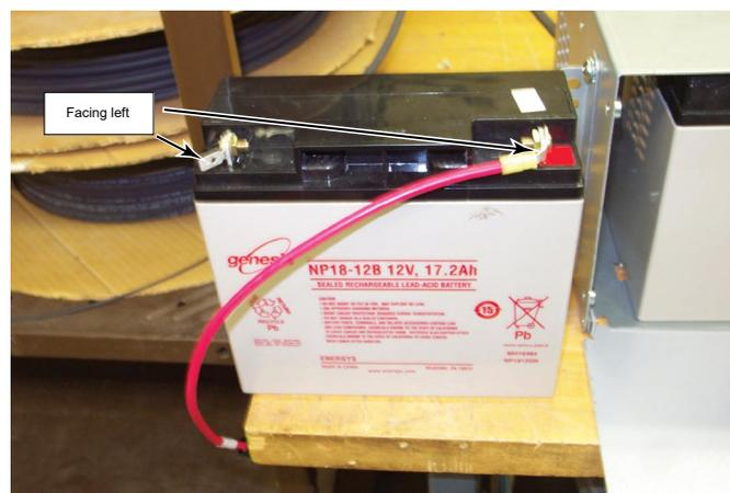
5. Set first battery in cabinet and attach the long lead (fast-on connector side marked positive) from the cabinet to the fast-on terminal on the positive terminal of the battery. See **Figure 24**.
