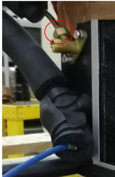
**Figure 2-5 Copper pipe connection inspection**
