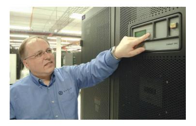
The Liebert FPC brings power distribution closer to the load, dramatically reducing the amount of cable needed to distribute power from the UPS. It also provides flexibility to change and add electrical distribution in the future.
